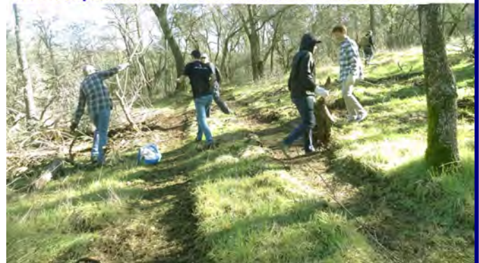
Over 80 volunteers drag the cut-branches on the *new* Center Trail uphill about 150 feet, to the *original* Central Trail (that will later be abandoned), using these cut-branches. Notice the two caterpillar tracks of the State Parks trail machine.
